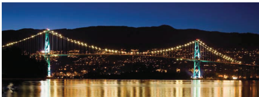
Lion's Gate Bridge, Vancouver
